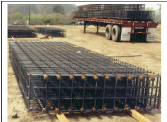
Fig. 1. BauGrids® as Shearwall Reinforcing
