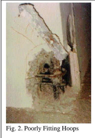
Fig. 2. Poorly Fitting Hoops
