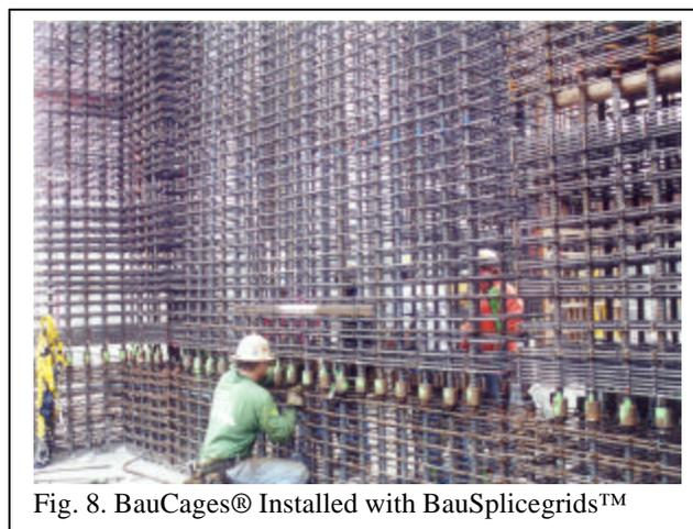
Fig. 8. BauCages® Installed with BauSpliceGrids™
