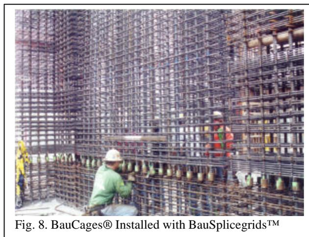
Fig. 8. BauCages® Installed with BauSpliceGrids™
